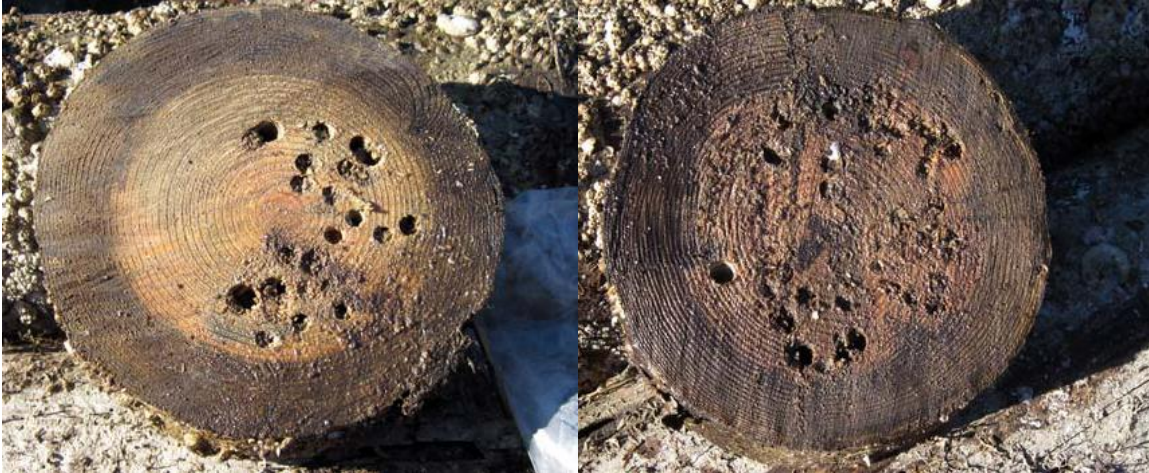
Figure 5. Sections of Two Piles Cut for Laboratory Testing
